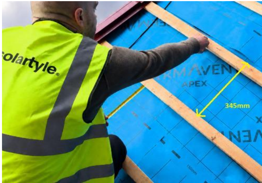
Batten spacing at 345mm centres shown with PermaVent Apex underlay
