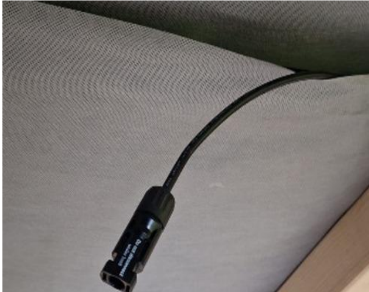
String cable routed through roof felt — ensure cable is protected and neatly positioned
