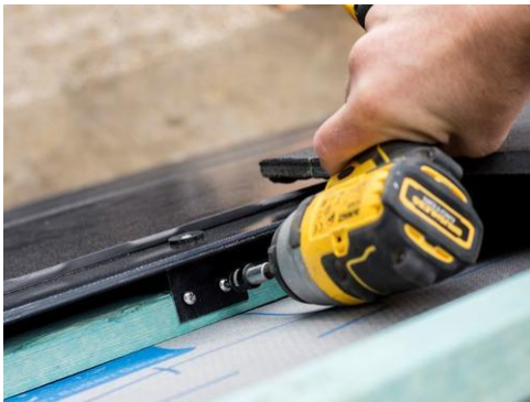
Fixing hooks into batten with screws
