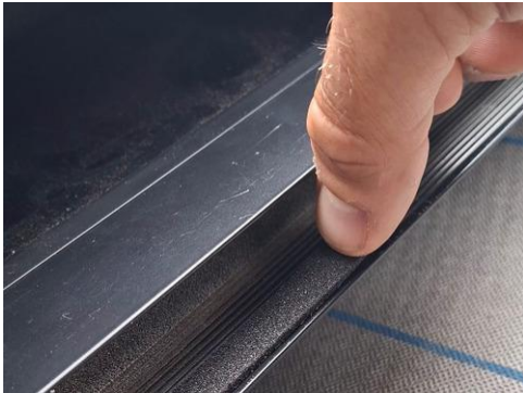
Apply the Compriband tape to the joiner channels
