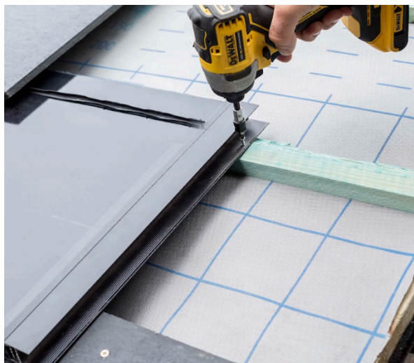
Securing joiners with fixings
