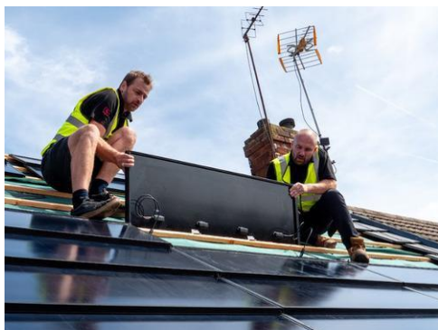
Left-to-right installation in progress
